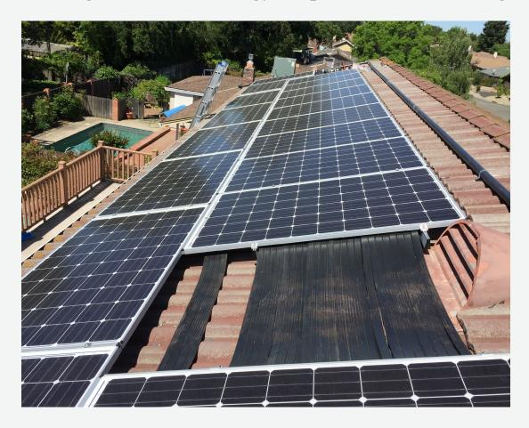
The Enertopia Glazed HEAT EXTRACTOR can capture heat independently from the solar panels, greatly enhancing the amount of energy available for process applications like mining, agriculture, industry. Below residential application for cooling PV panels and heating swimming pool using unglazed Heat Extractor.
