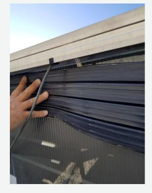
In order to couple the panel to the recyclable flexible elastomer device and not shock the panel or break the glass, Enertopia has developed a breakthrough technology that acts like a thermal check valve allowing heat to go one way on the back of the panel
